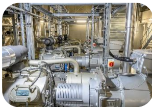
Sabroe compressor repairs parts
